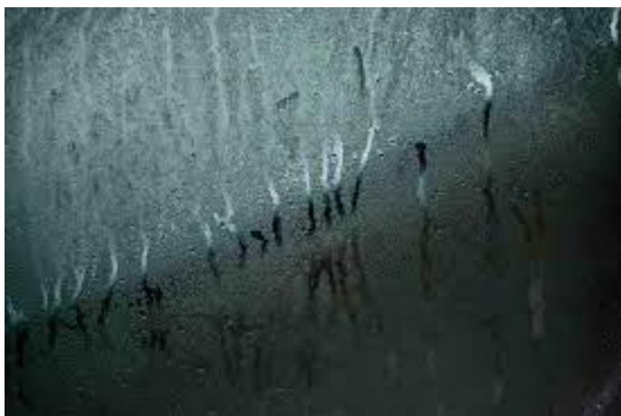
Pic 13: Condensation on glass.
