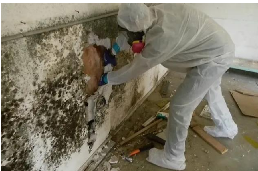
Pic 5: Removing contaminated material.
