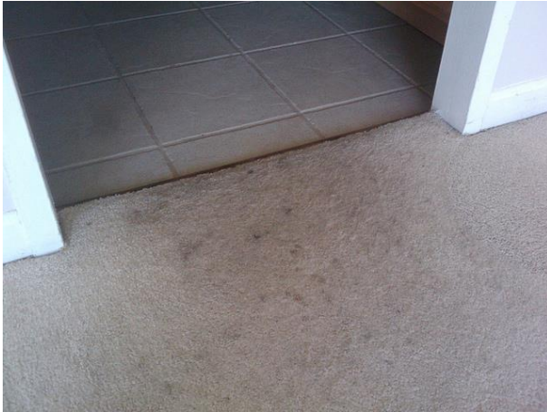
Pic 9: Mold growth on carpet.
