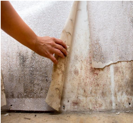
Pic 12: Mold growth under wall paper.
