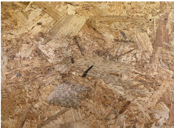
Pic 6: Mold growth on wood.
